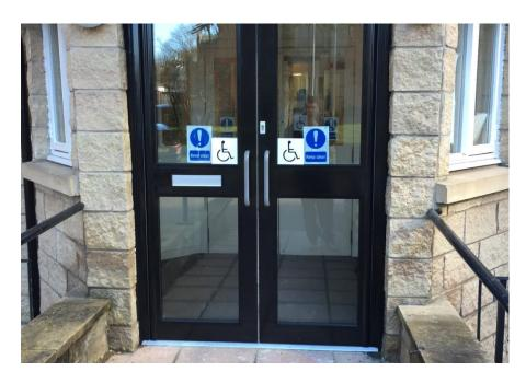
Debridge Doctor's surgery in Bearsden in Scotland. This is a record DFA 127 FULL POWER door. As this door has a programmable micro-processor the speed of opening and closing can be adjusted.
