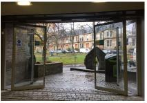
This record Total Opening System (TOS) was installed at the entrance to the Geographical and Earth Sciences department at Glasgow Caledonian University. The TOS system allows these sliding doors to be released to provide the widest possible escape route in the event of an emergency.
