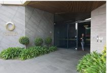
For this twin sliding door entrance at 2-4 Yarra Street in South Yarra, record Automatic Doors replaced the existing sliding door operator to the external entrance, due to continual breakdowns and unreliability, with an STA 22 heavy duty operator.
