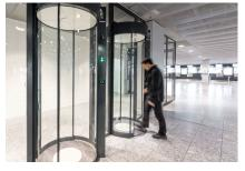
Security is an essential issue for an airport. This is also the case at Zurich Airport. In order to ensure a secure separation between the Schengen and non-Schengen areas and still allow staff to pass through them, two new record R 62 security interlocks were installed. The high flow rate as well as the reliability are an essential criterion for the choice of the product for the airport.
