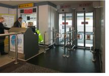
This record FlipFlow WIDE extended is installed at Glasgow International Airport. The units can be operated singly and so not used when not needed. The FlipFlow system allows safe and secure passage of persons into or from areas where security is a priority and a controlled flow of people is required.
