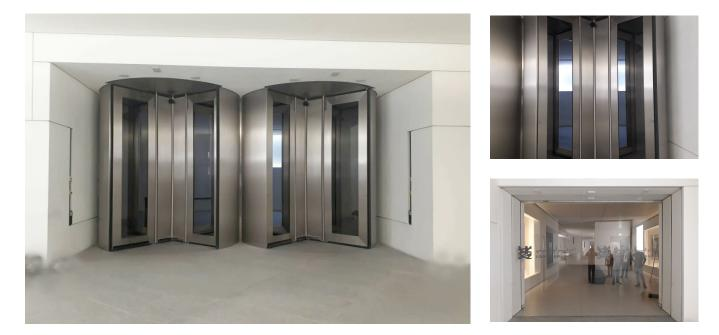
Automatic revolving doors type record K 41 V32 in stainless steel cladding 316 brushed finish with a diameter of 3'290 mm and a total height of 3'150 mm.
