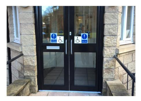
Debridge Doctor's surgery in Bearsden in Scotland. This is a record DFA 127 FULL POWER door. As this door has a programmable micro-processor the speed of opening and closing can be adjusted.
