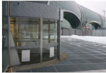
record K 21 revolving door with integrated sliding door
