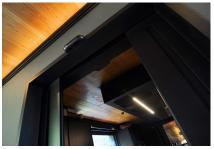
Automatic sliding doors record STA-20 installed by the entrance to the kitchen and to the gym. To emphasize the architecture of the stone wall by the main entrance, the operator record STA-20 was mounted between the wall and the ceiling.
