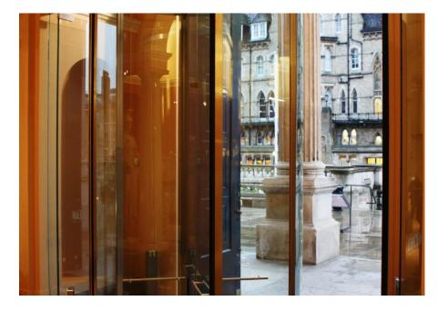
This entrance to the Ashmolean Museum in Oxford is fitted with a record K41 four wing revolving door. Revolving doors can also have larger diameters and curved sliding doors. Larger models can have display cabinets internally.
