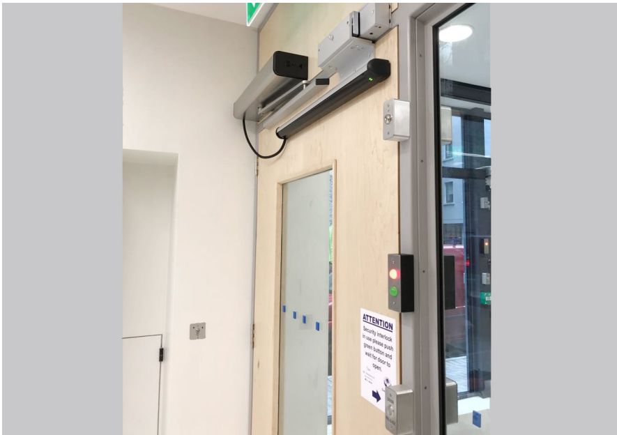
record DFA 127 swing door with interlock system
