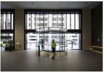
For the York Street lobby entrance of the Dexus owned 26 storey commercial office building at 44 Market Street Sydney, a 4000mm diameter record Diamond Series revolving door was installed as part of significant building refurbishment works undertaken by Growthbuilt and designed by Wood Bagot.
