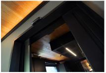
Automatic sliding doors record STA-20 installed by the entrance to the kitchen and to the gym. To emphasize the architecture of the stone wall by the main entrance, the operator record STA-20 was mounted between the wall and the ceiling.
