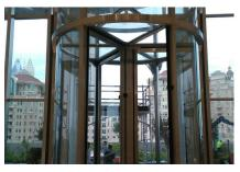
Revolving door record K31 with invisible under floor drive. size 4'400x6'000 mm
